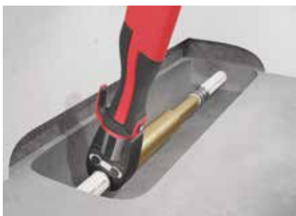
Fig. 29: Installationstrin, reparationskobling.
