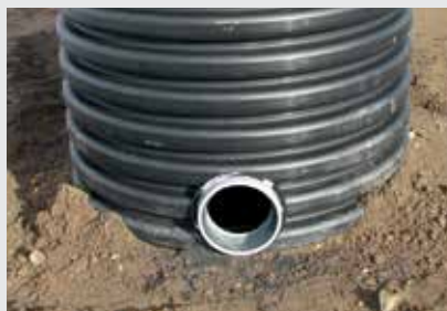
5. Lubricant is applied to the inside of the installed seal, allowing the socket fitting to fit into it.
