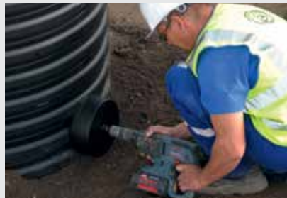
2. The edges of the opening are then deburred.
