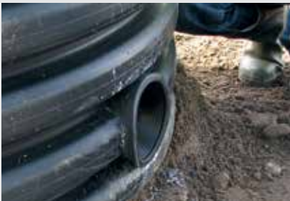
4. If installation is difficult, the edges of the hole can be coated with lubricant.
