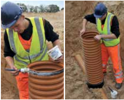
10. Lubricate the gasket on the riser pipe and press the riser pipe into the chamber base socket.
