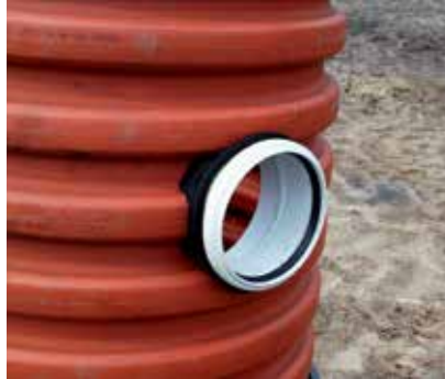
5. Lubricant is applied to the inside of the installed seal, allowing the socket fitting to fit into it.
