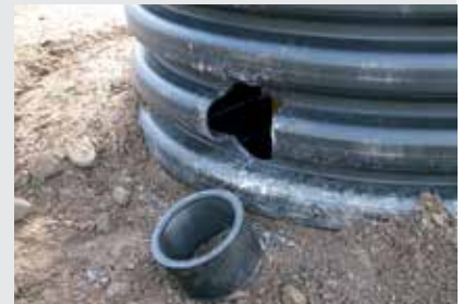
3. The in situ insert seal is mounted in the hole made.
