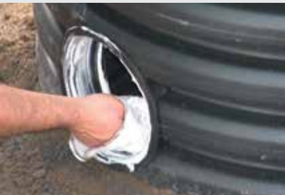
1. A hole is made in the corrugated tube with a special jigsaw.
