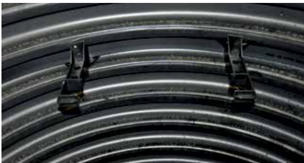
Fig. 5. Pre-assembly of the ladder clamp in the riser pipe
