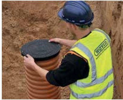
11. Secure the chamber to prevent the entry of sand while filling the excavation.
