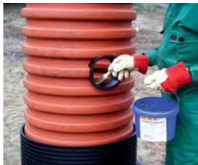
2. The edges of the opening are then deburred.
