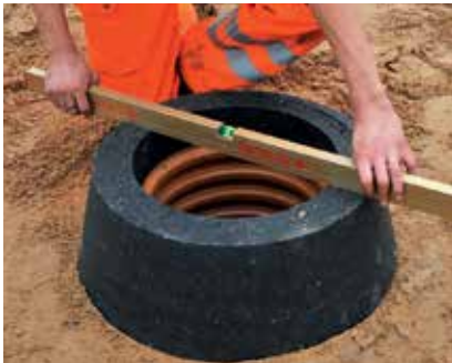
13. Install one of the recommended chamber tops.
