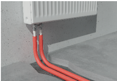
Fig. 47: Radiator installation examples with “Eurocone” screw connection.
