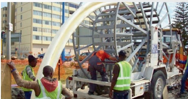
South Africa, Durban, DN250, sewer rehabs
