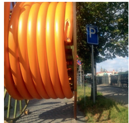
Prag, City, DN500, SDR 17, trenchless rehabilitation, Zepris s.r.o.
