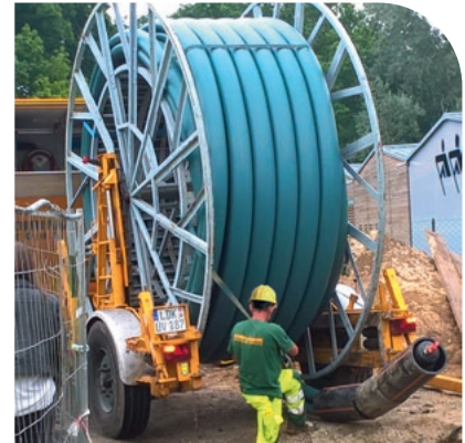
Wolfsburg, Allerpark / VFL stadium, Wastewater, DN300, SDR 17, trenchless rehabilitation, Diringler & Scheidel
