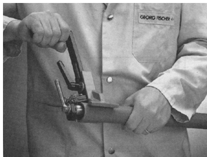
Chamfering the pipe.
