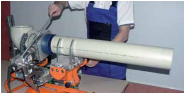
fixing and aligning the components, then heating them up
