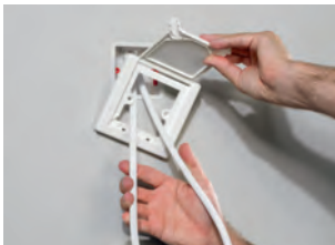
Figure 53: Installation procedure of HX113 cover plate
