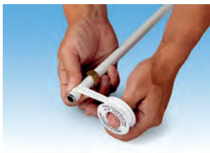
Apply PTFE tape if required
