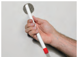
Figure 22: Always protect pipe ends
