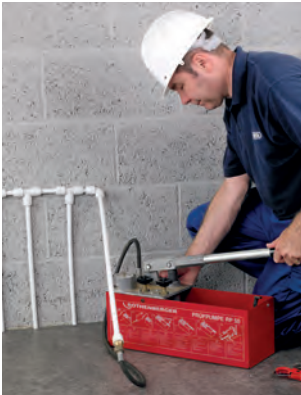
Figure 60: Pressure testing
