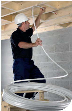
Figure 23: Packaging retains pipe until last metre
