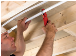
Measure and cut in-situ
