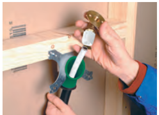
Figure 50: Installation of HX102 terminal fitting plate and HX101/15, 15mm conduit terminal
