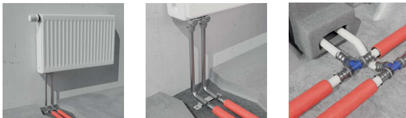
Fig. 47: Radiator installation examples with angle connection pipes.
