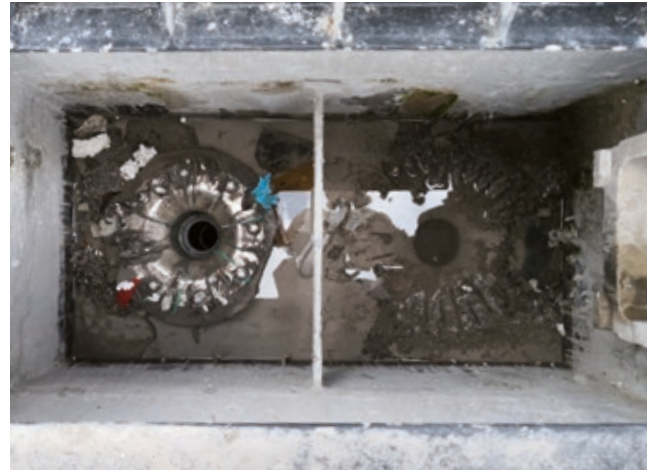
Figure 63: Periodically maintenance to roof outlets
