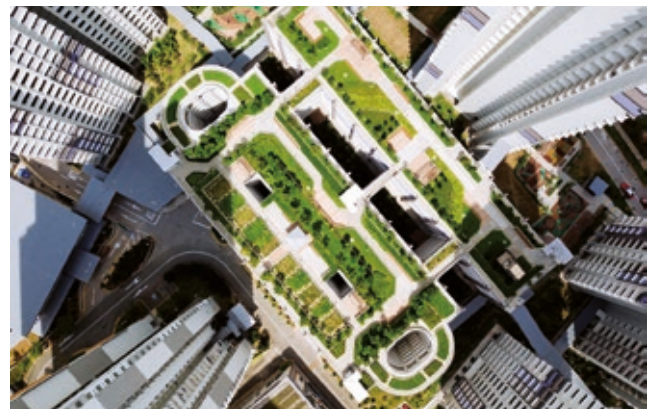
Figure 9: Rooftop, The Hague
