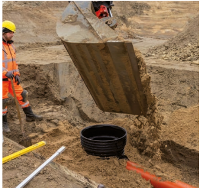
Figure 52: PVC pipe installation
