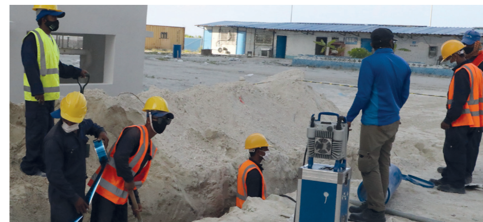
Construction of water and sewer network, The Maldives.
