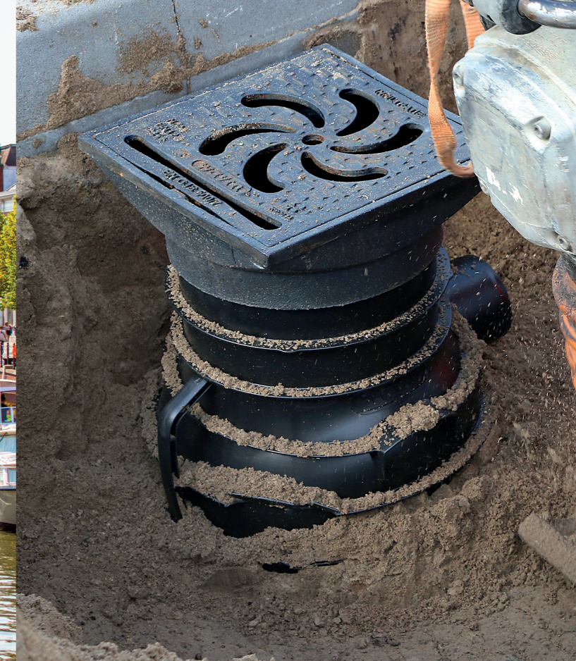
Installation of a Tegra Road Gully.
