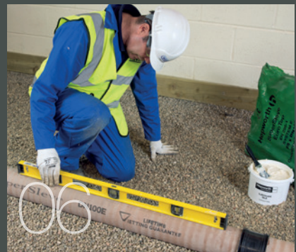
06 Check the pipeline is laid to the correct gradient
