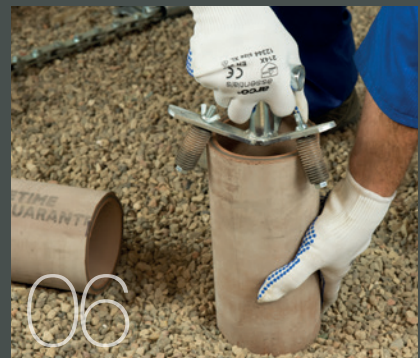
06 Remove any sharp edges with pipe trimmer
