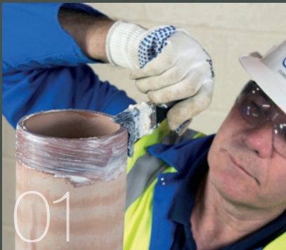
01 Lubricate the pipe end
