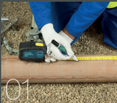
01 Mark the pipe to be cut
