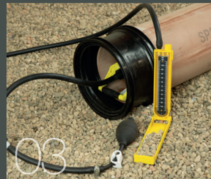
03 Connect a "U tube" gauge (manometer) to the testing stopper
