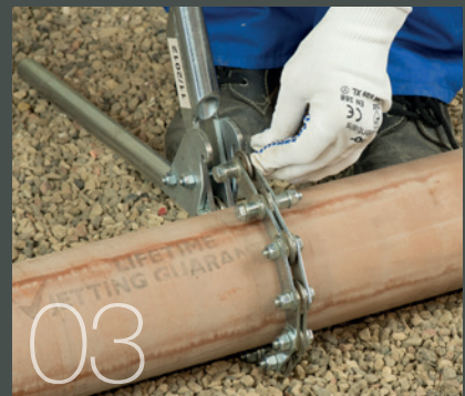
03 Hook the chain onto the jaw of the pipe cutter
