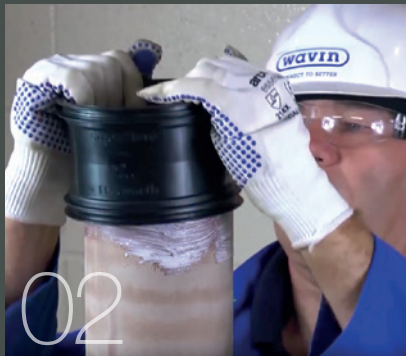
02 Press the coupling on to the lubricated pipe end
