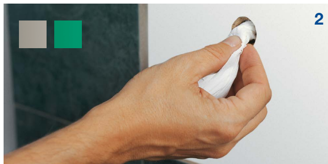
Dry and degrease. Measure and mark the depth of insertion on the stake depending on the wall thickness of the drilled through pipe + 2 mm; set the distance ring on the heating adaptor.
