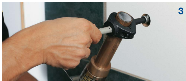
Start heating the repairing stake and adaptor and insert the heating stake slowly and without turning into the prepared hole. Heat for 5 seconds.
