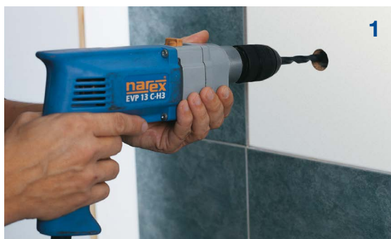
The drilled hole must be redrilled (calibrated) with a 10 mm drill.
