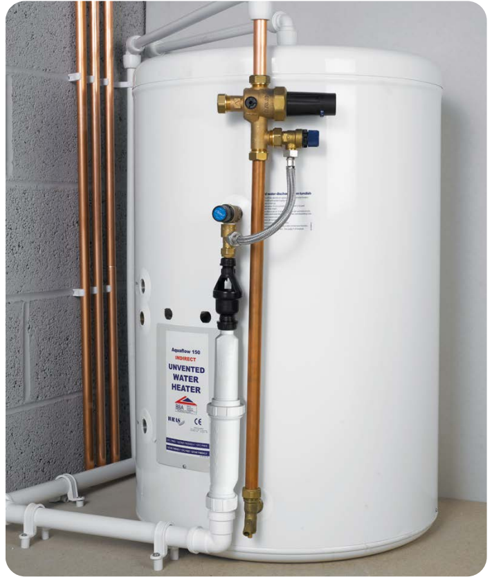
Fig 6 Self-sealing valve when used with a combined temperature and pressure relief valve for unvented hot water storage system.
