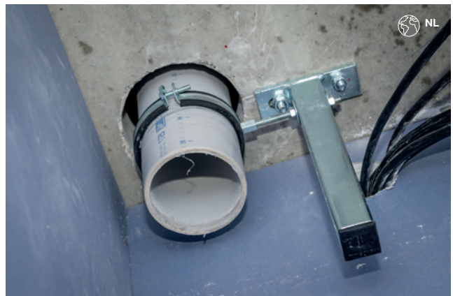
Figure 11: Fastening to elements containing mass
