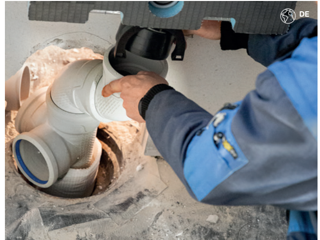
Figure 42: Setting up a sewage system for a floor slab
