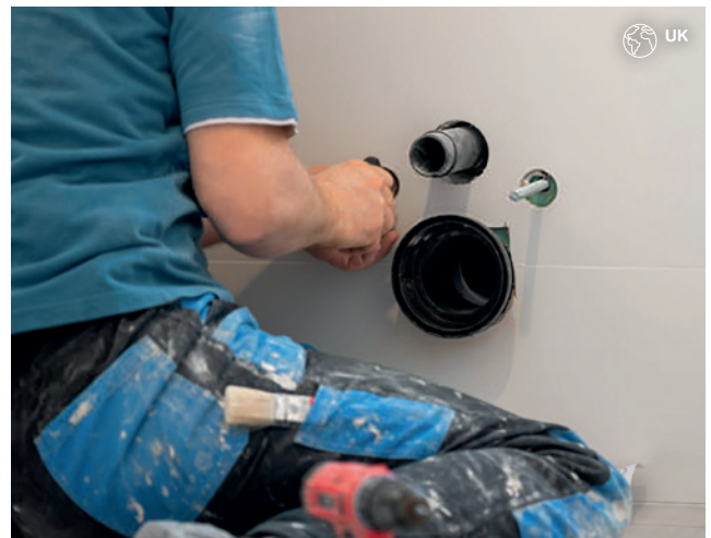
Figure 43: Installation preparation for the ceramics
