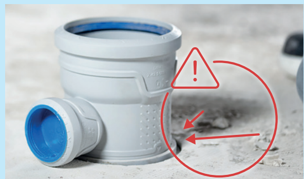
Figure 21: Building debris as a structure-borne sound bridge
