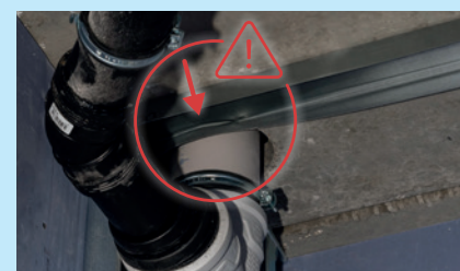
Figure 41: Avoiding contact with profiles
