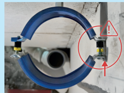
Figure 40: Aligning the pipe brackets correctly
