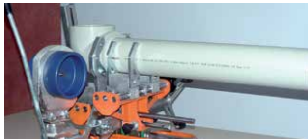
finished weld after the cool-down
