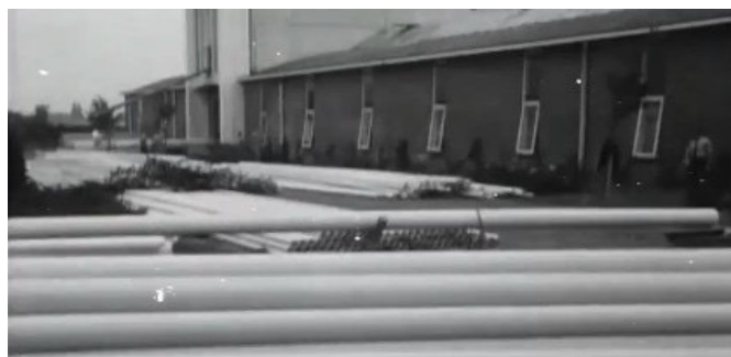
Fuente: "PVC Pipe Longevity Report – A Comprehensive Study on PVC Pipe Excavations, Testing and Life Cycle Analysis". Buried Structures Laboratory, Utah State University. Mayo 2014
