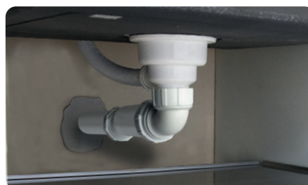
Membrane opens and closes, to prevent foul sewer odour from returning.
